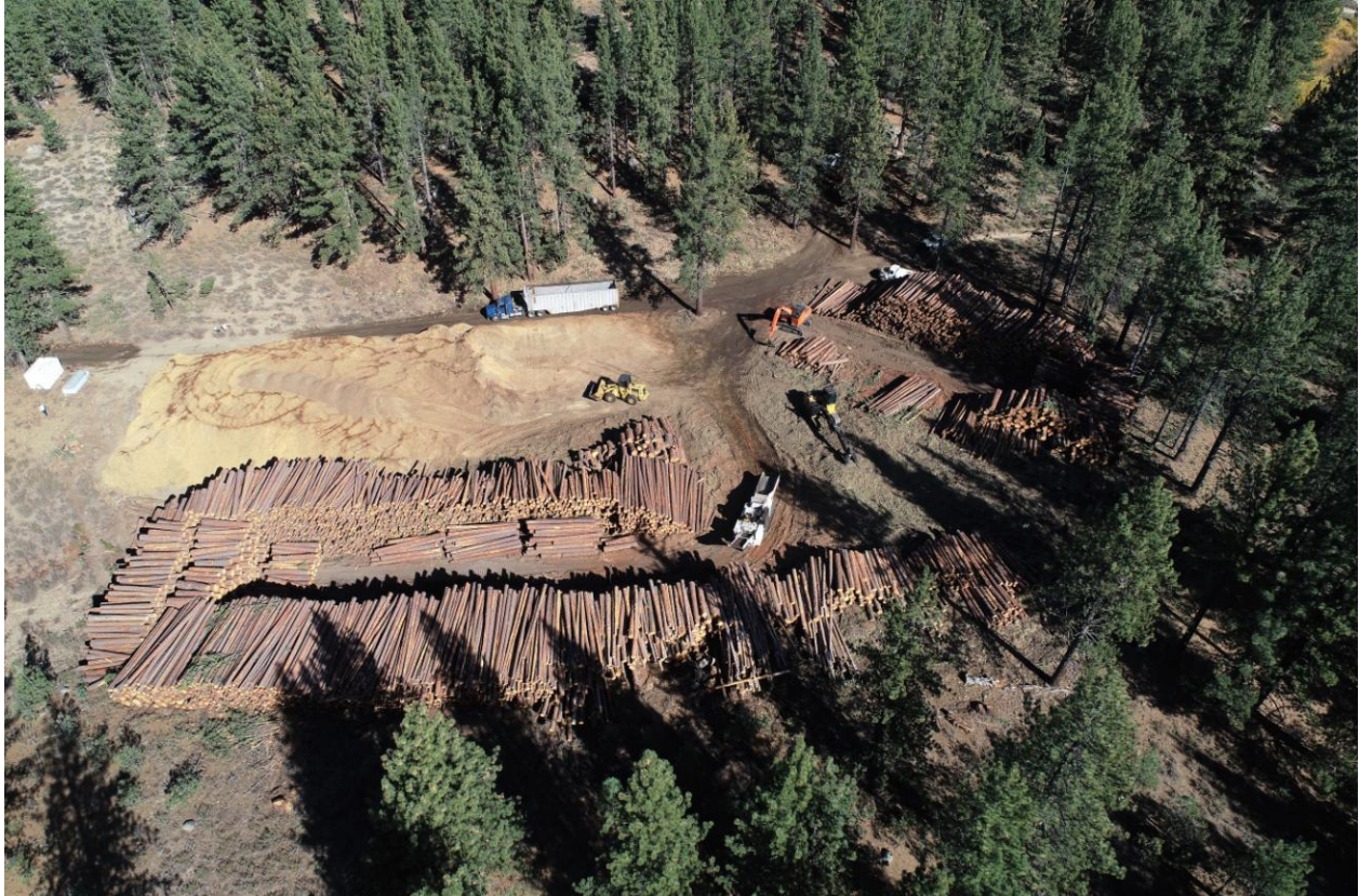
Markit! Forestry's log landing for the Spooner Lake Landscape Restoration Project
